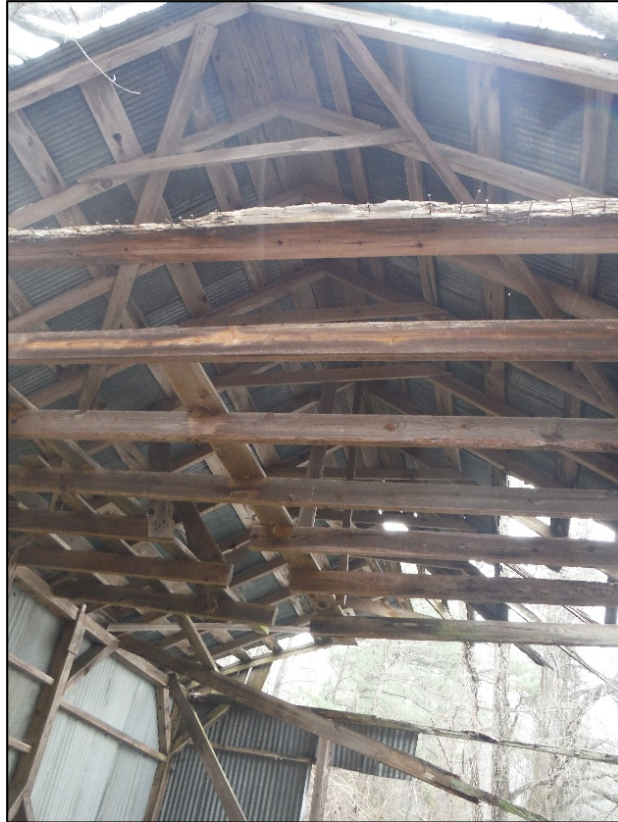
Figure 8. View of the McCallum Mill building (MG0153), rafters, facing north.
