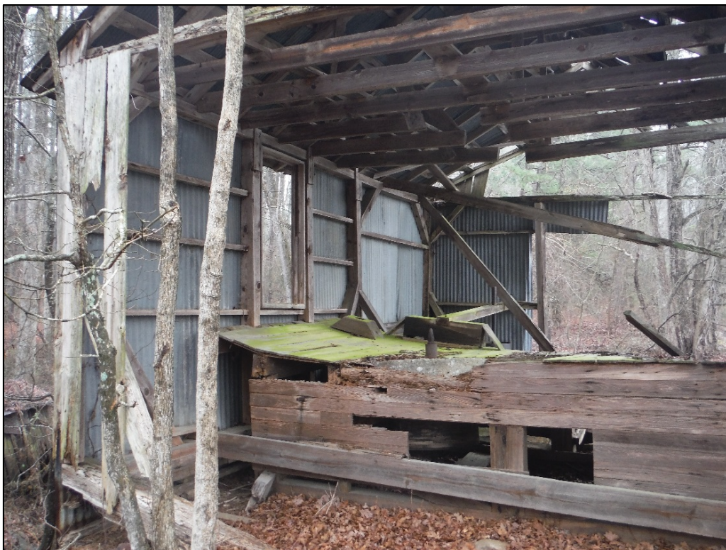
Figure 9. View of the McCallum Mill building (MG0153), interior, facing northwest.
