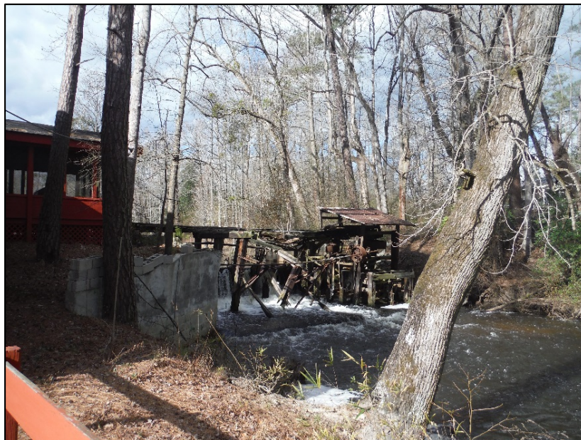
Figure 28. McNeill's Mill (HK0016) dam and mechanical equipment, facing west.
