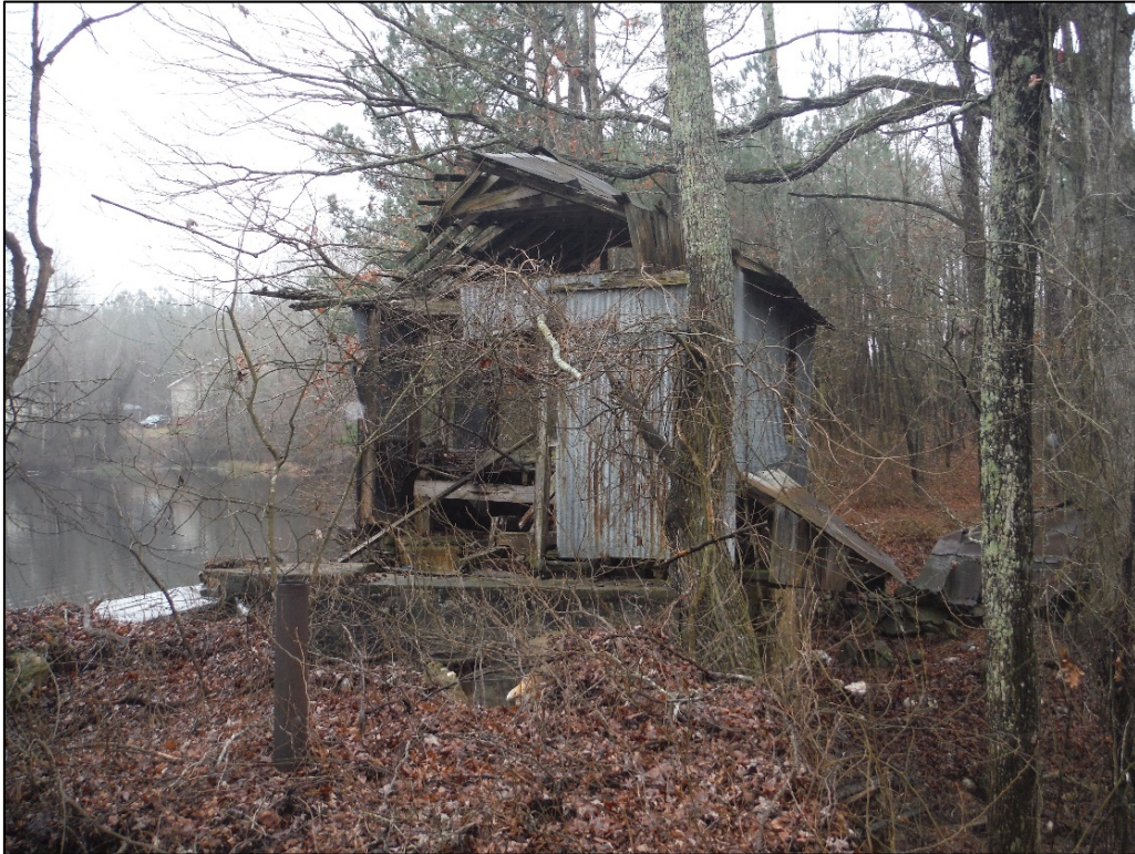
Figure 6. View of the McCallum Mill building (MG0153), facing south.
