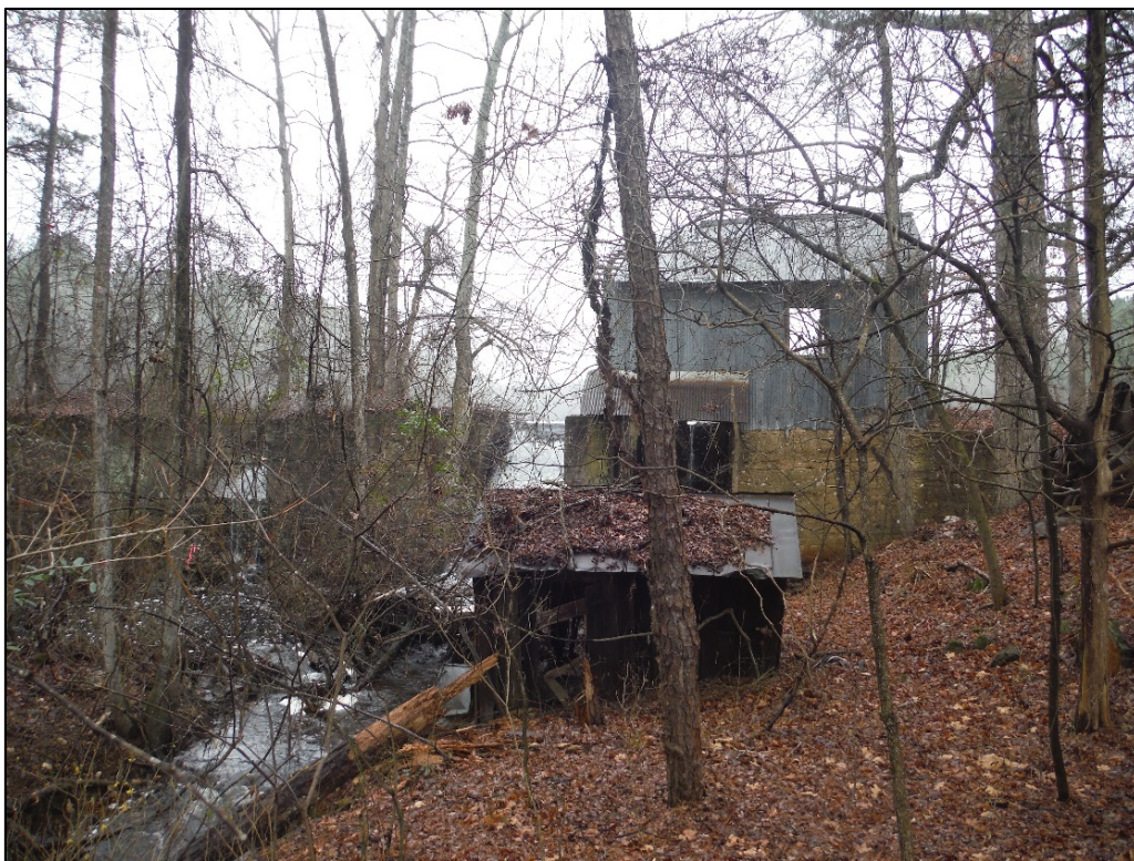
Figure 3. View of McCallum Mill (MG0153) (PIN 757500081325), facing east.
