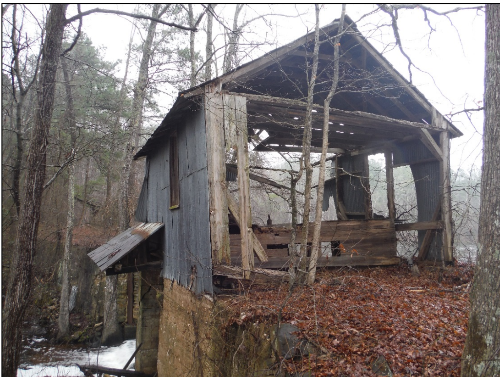
Figure 7. View of the McCallum Mill building (MG0153), facing north.
