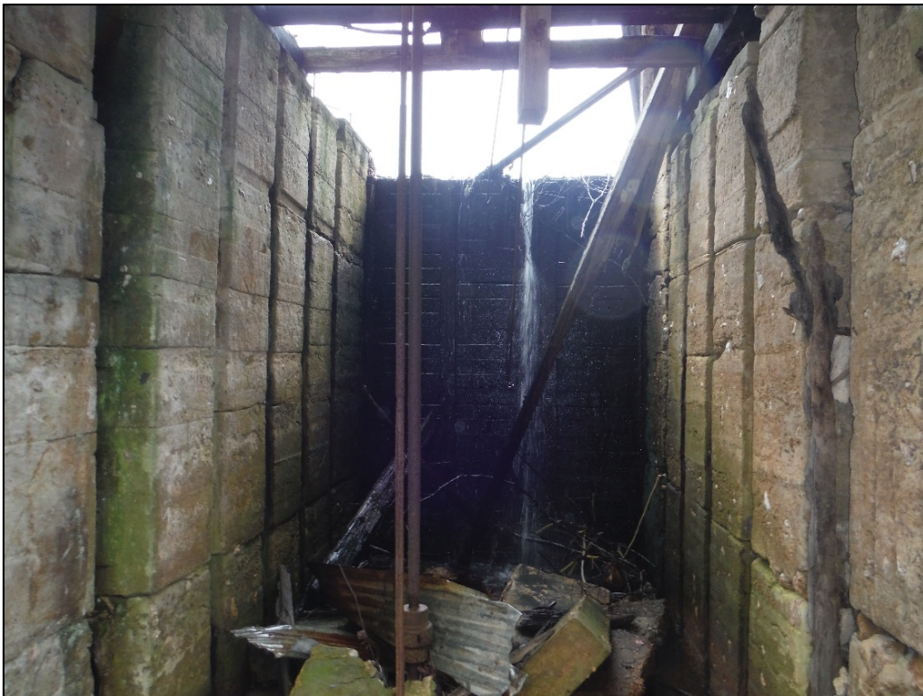
Figure 11. View of the McCallum Mill building (MG0153), millrace, facing east.
